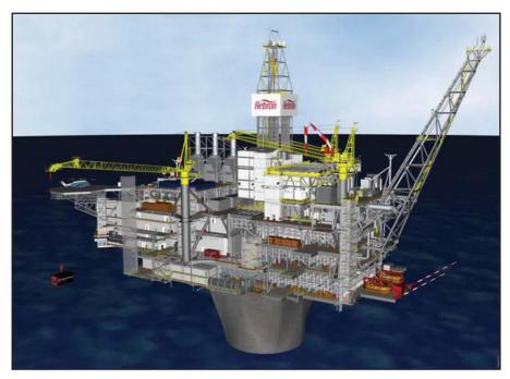
$The \ reinforced\ concrete\ GBS\ supports\ the\ topside\ modules, like\ drilling, housing\ and\ power\ generation\ modules.$
