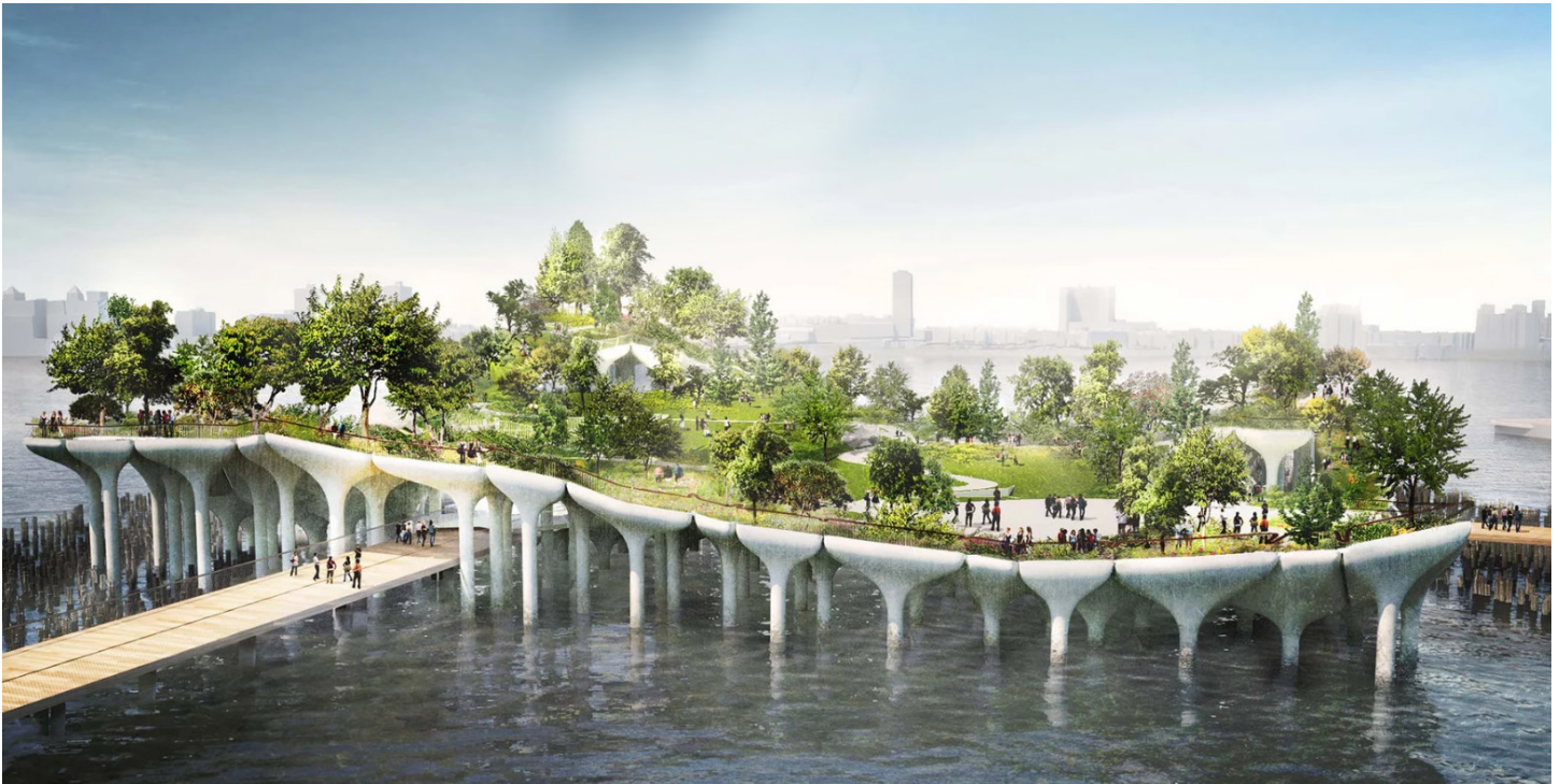
This rendering shows to concrete "Tulip Pots" used to support the structure.
